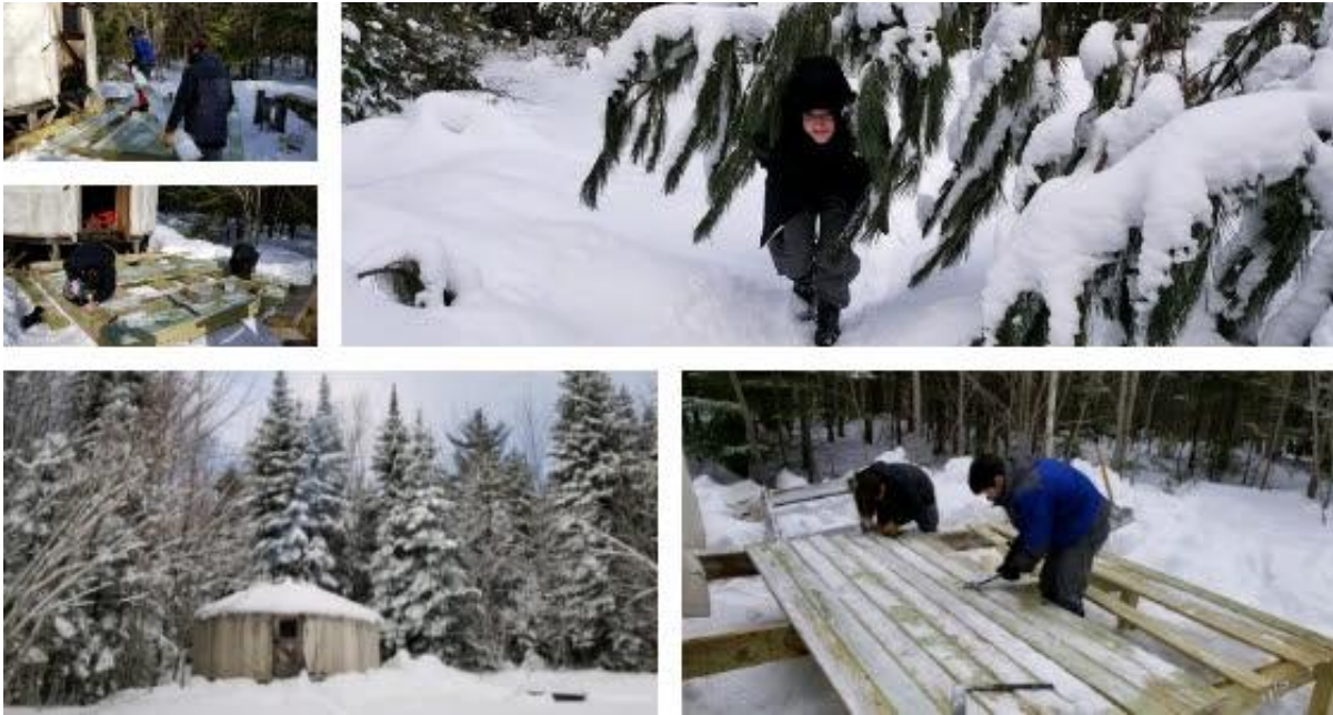
Working on building the decks for the yurts.
